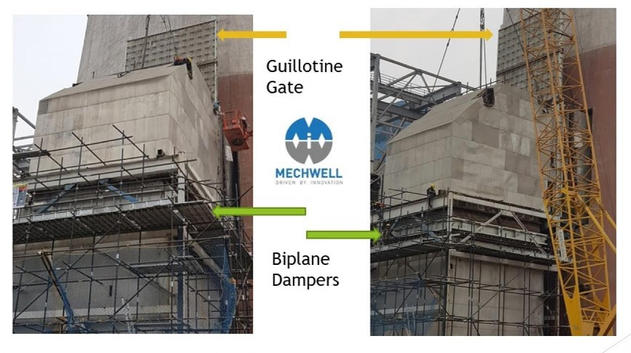
Image Showing Guillotine Gate being installed at Site in vertical position and Biplane damper being installed in horizontal position for FGD System at 3x500 MW IGSTPP JHAJJAR -
