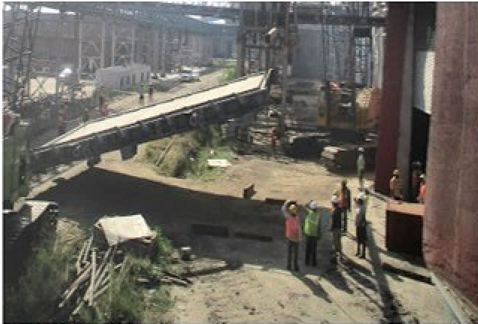
DAMPER LIFTING AT SITE
