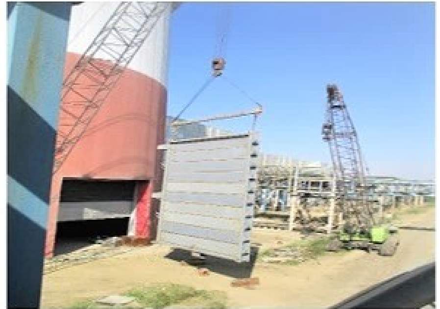
Vertical Position Of Damper
